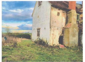
Another early job was taking off all the existing external wall covering as it was virtually all cement. Cement render on a timber frame building is the 'kiss of death' to the integrity of the timbers. Cement does not allow the building to breathe so the timbers underneath get wet, stay wet, then rot slowly. Some of the sections of cement, were about 4 inches thick and reinforced with rusty metal mesh. This was a difficult, dirty, and potentially dangerous job.
