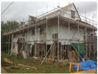
As soon as the main structural timber work had been done, we moved our attention to the roof. Initially we thought it would be sufficient to merely repair the section with the hole in it. However, we finally decided to redo the entire roof. We organised full scaffolding and then started to carefully remove the old peg tiles. We managed to save, clean, and reuse well over half of the original tiles and then had to make many trips
