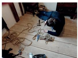
help, putting rope in the gaps between the new floorboards in the first-floor lounge area, a job called caulking.
